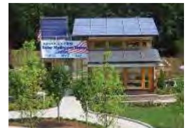
Renewable Energy Storage
